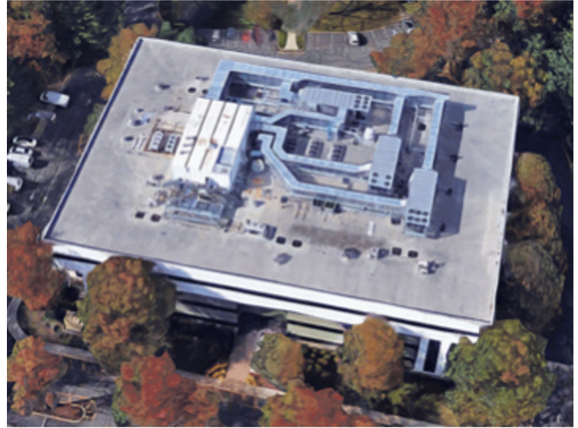
Building to reconstruct
